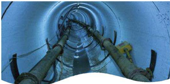
Above: Internal view of the curved portion of the Homestead Avenue Interceptor Extension installed using trackless pipe tunneling technology, which represents the first time this has been completed in the U.S. Below: MDC, AECOM and NE Remasco staff stand above the receiving pit where the tunnel boring machine broke through right on target.
